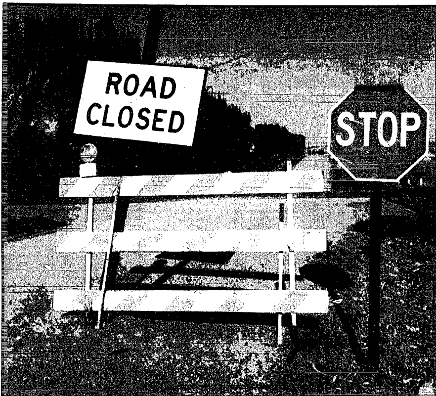
Roadblocks, caution signs and road-closed signs went up along state Highway 15 this spring. Photography: Randall Howell
